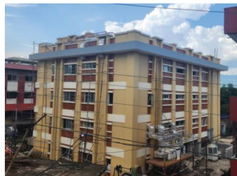
Figure 3: OT block in Bhaktapur Hospital
